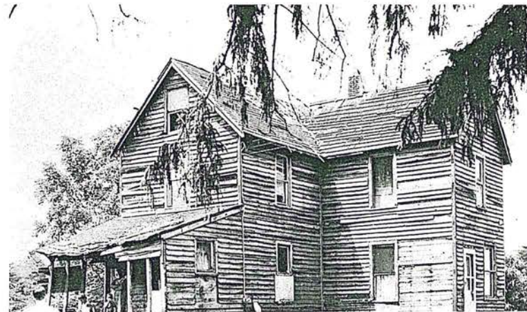
This eerie-looking structure was the home of one of the families who built a new home under Farmers Home Administration self-help program.
