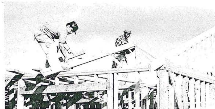
Installing roof trusses . . . part of the six family group in Kingsburg, California.
