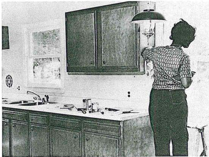
Mother working on kitchen cabinet in one of the self-help homes built under the Farmers Home Administration program, Cumberland County, New Jersey.
